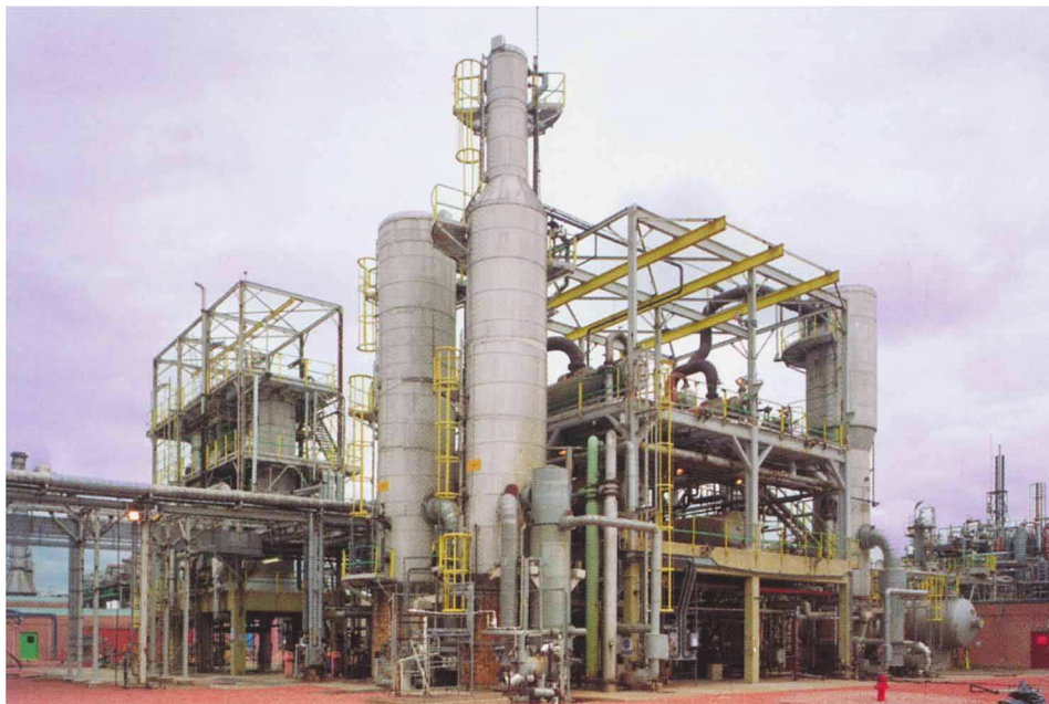
Figure 2.8 Industrial fractionating columns used in an oil refinery.
