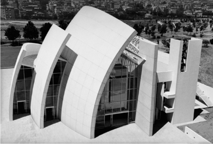
Fig. 29.10. The church of Dives in Misericordia , in Rome, built with a photocatalytic cement (Italcementi). Architect: Richard Meier
