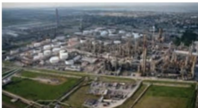
Fig.9: A chemical plant
