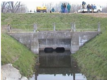
Figure 20. View of the Hatarmenti water-gate
