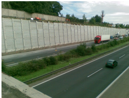
Figure 18. Situation before final completion of the works
