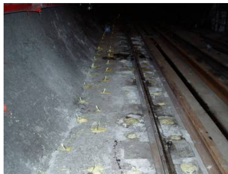
Figure 32. View of the railway after repair works
