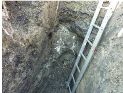
Figure 21. Grouting material in the surrounding of the water-gate (photo from the control excavation after 10 years)
