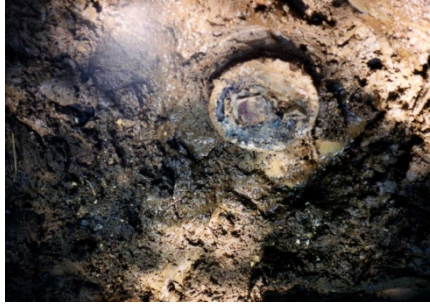
Figure 22. Borehole with contaminated water seepages
