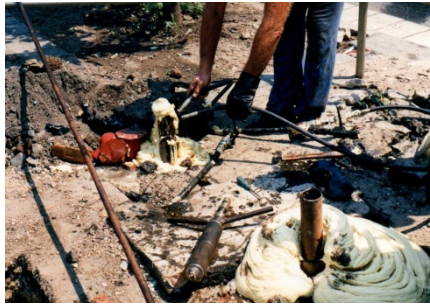
Figure 23. Sealing of the borehole with PU grouting
